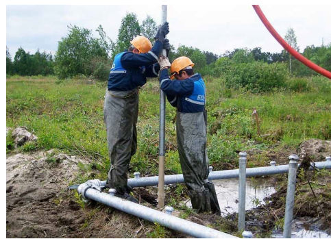
On-site equipment handling
