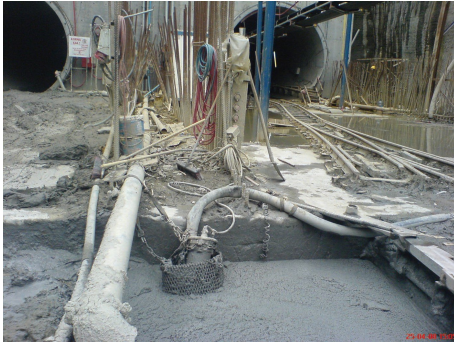
Excavation and site pumping
